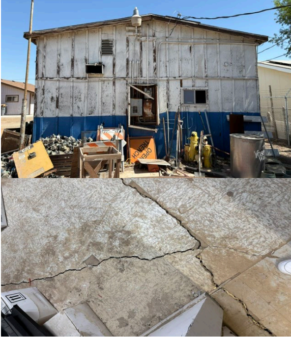
Shop & Storage Building Repairs
