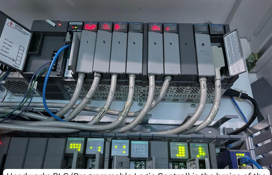
Headworks PLC (Programmable Logic Control) is the brains of the automated system that controls the equipment. This also sends out alarms in cases of emergencies or breakdowns.
