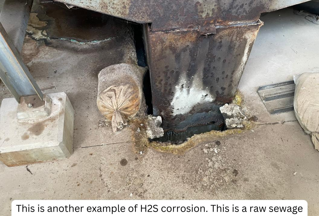
This is another example of H2S corrosion. This is a raw sewage drum screen foundation. This foundation is being corroded by constant H2S gasses.
